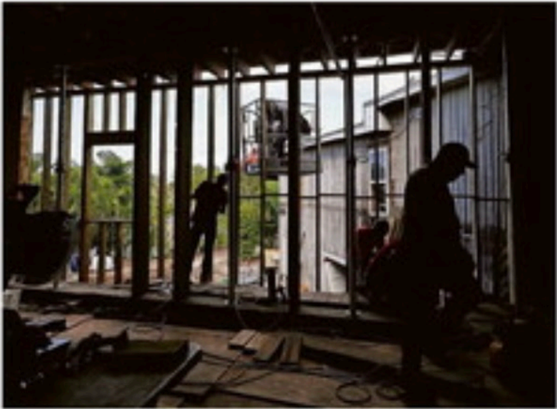
Laborers re-frame a wall during the renovation process at the historic Collier Inn on Useppa Island on Oct. 7. RICARDO ROLON/USA TODAY NETWORK - FLORIDA
